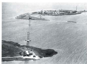
Construction of the first cable car to the island, 1926
